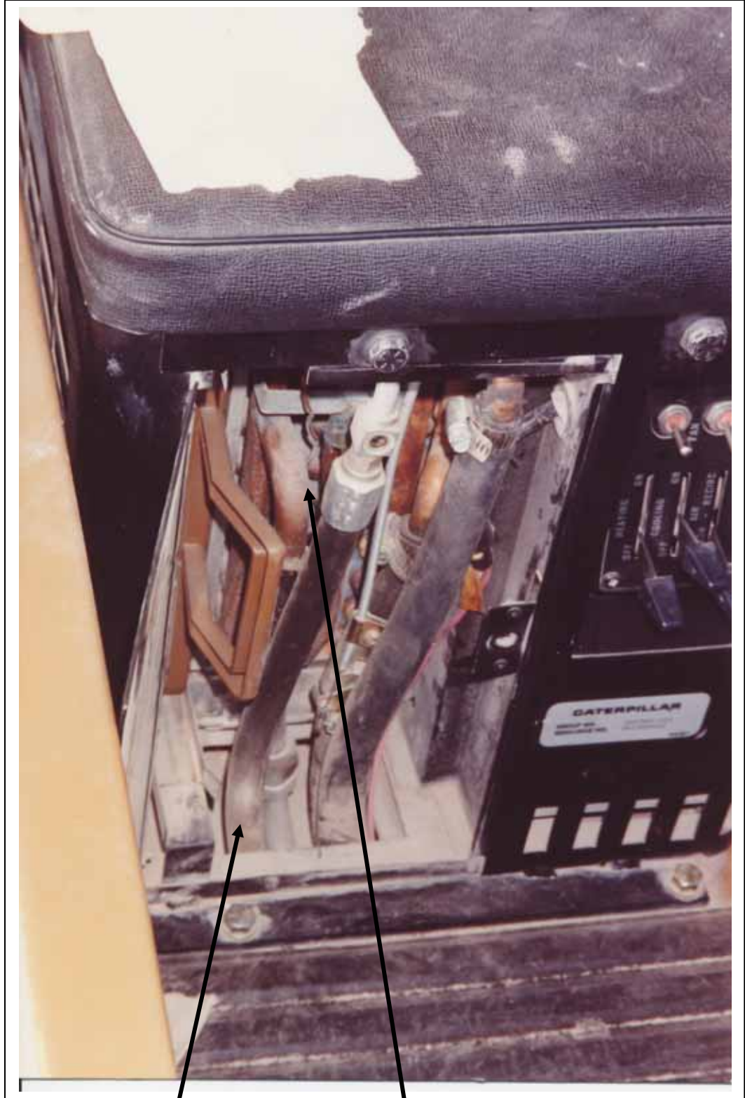
Hose coming up through floor. Run clutch wire here as well.
