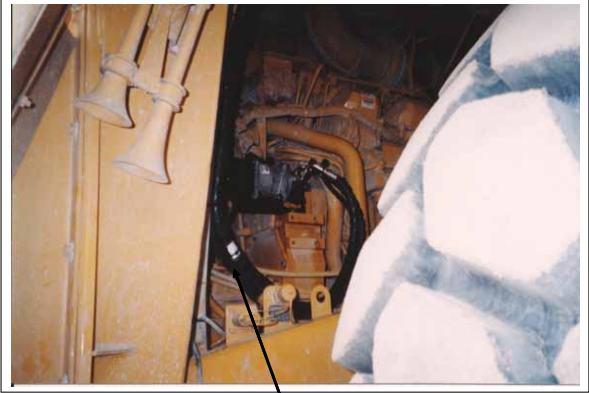
Hose runs and clutch wire running to condenser and cab.
